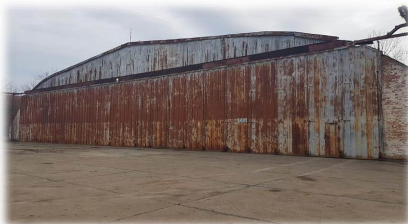
Figura 18 – Imagini imobil C24 - Hangar
